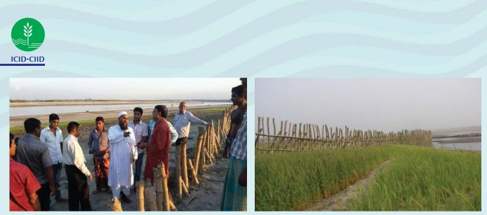
Figure 4(a): River bank sedimentation (3.5 m) instead of erosion; Figure 4(b): Crop production in place of river bank erosion [The officials of the BCCTF are visiting the performance of the bamboo bandalling structures constructed in the Old Brahmaputra River near North Sirajabad of Islampur Upazila under Jamalpur District The BCCTF officials are visiting the project site (left) and bumper wheat crop cultivated in the bank protected area (right)]
